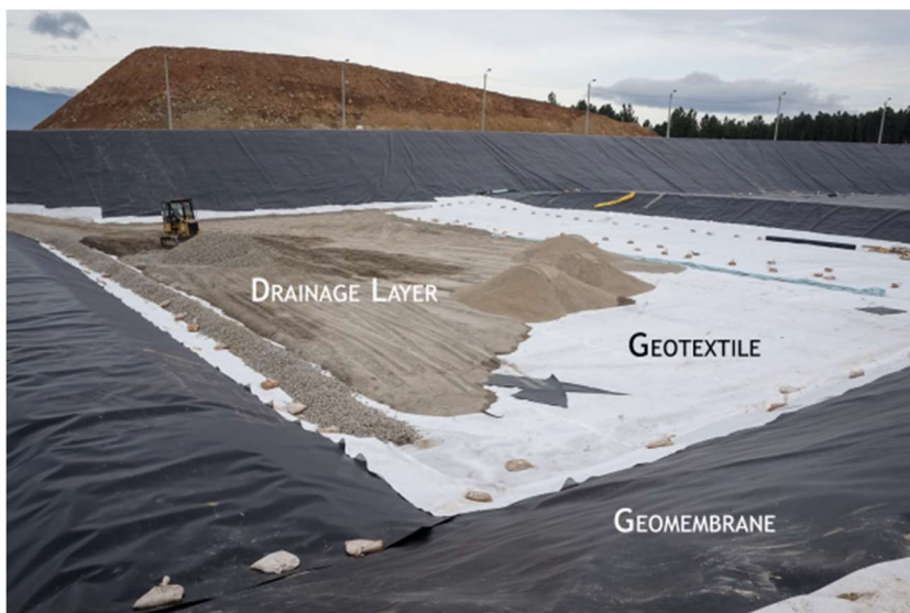
Base liner system of a waste landfill.
