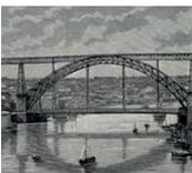
Projected by the engineer Teófilo Seyrig, a disciple of Eiffel, it was inaugurated in 1886 and is composed by two overlapping iron decks. The bridge is 395 metres long and 8 metres wide, and its arch is still considered to be the world's biggest created in forged iron.
