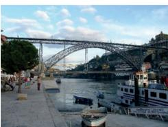
Planned by engineer Teófilo Seyrig, a disciple of Eiffel, it was inaugurated in 1886 and is composed by two overlapping iron decks. The bridge is 395 metres long and 8 metres wide, and its Arch is still considered to be the world's biggest one in forged iron.
